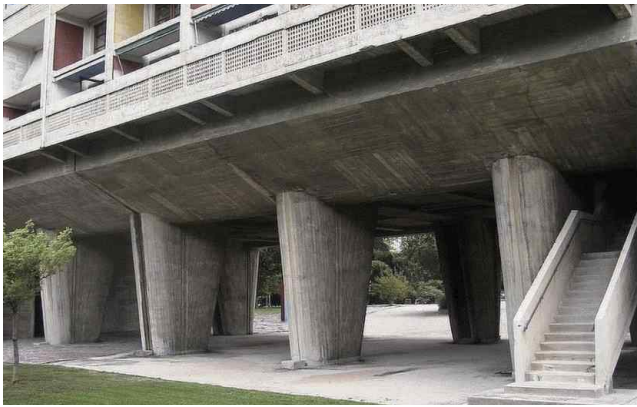
Figure 12. Exposed concrete exterior of Le Corbusier's Unité d'Habitation, Marseilles, 1947-53 (Author's photo)
