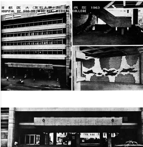
Figure 1. Soo-Do Medical College Hospital, Seoul, 1963-65, as published in SPACE (April 1968): The images were captioned “(Top left) Exposed Concrete Facade; (Top right) Ceramic Relief; (Bottom) Main Entrance and Canopy”.
