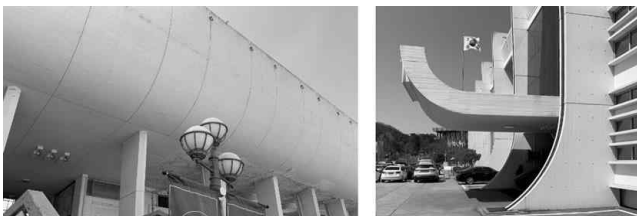
a) Northern entrance b) Southern entrance
