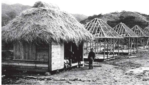
Figure 2. Prefab housing in Okinawa (1946) 59)
